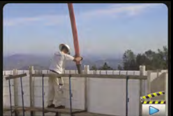
Concrete Placement
